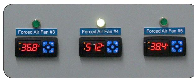
Figure 6. Sensors monitor “warm” air temperatures (°F) exiting the column of bins in the serpentine horizontal/vertical airflow system in Figure 4. At the time of this picture, cold air entering Forced Air Fan #4 was 35.6°F (2°C) and the internal temperatures of three individual, equally sized pears being monitored were 59°F (15°C), 67°F (19°C) and 68°F (20°C) along the cooling path, averaging 64.4°F (18°C). Fruit started at about 71.6°F (22°C), so the temperature at Fan #4 (51.2°F; 10.7°C) is about halfway between the cold air entering at 35.6°F (2°C) and the average internal temperature of cooling fruit at 64.4°F (18°C). With experience, one can make good predictions about internal fruit temperatures at any time within the bins. (Photo by Hugh W. Fraser, OMAFRA)
